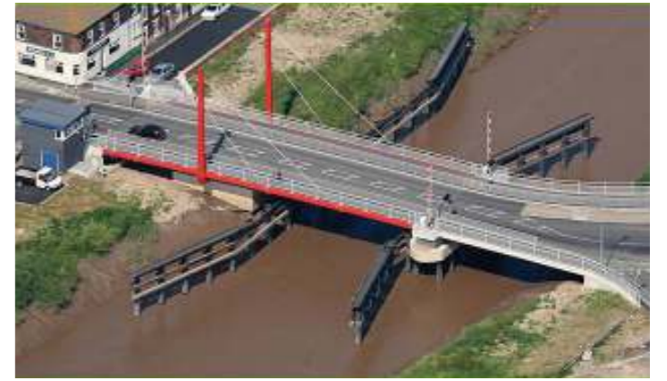
Dutch River Swing Bridge, Gooles.
