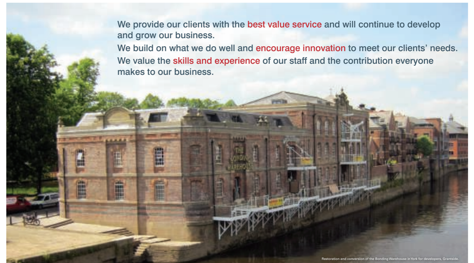
Restoration and conversion of the Bonding Warehouse in York for developers, Grantside.
