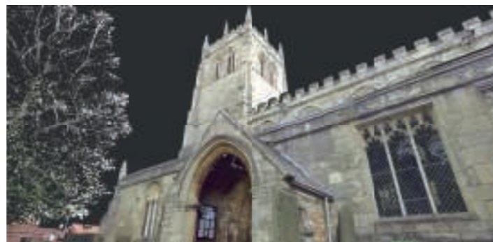
St Cuthberts Church - Point Cloud
