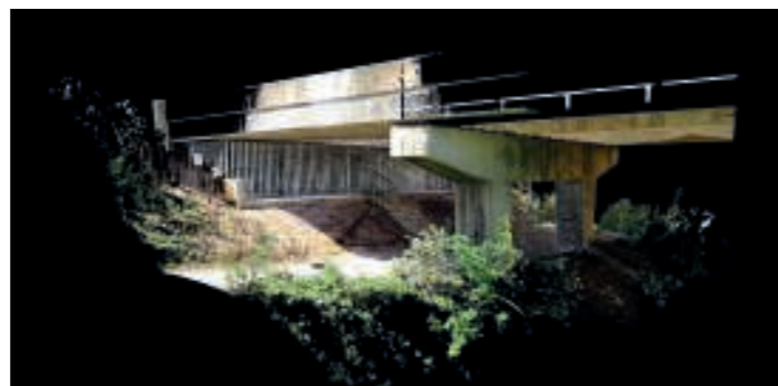
Tickton Flyover - Point Cloud
