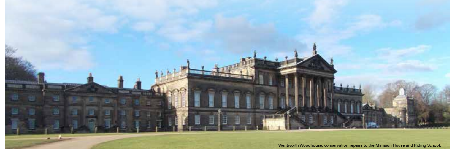
Wentworth Woodhouse: conservation repairs to the Mansion House and Riding School.
