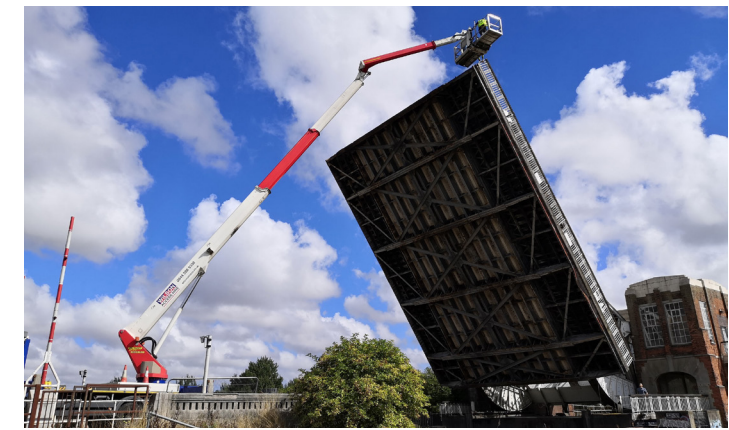
Sutton Road Bridge Hull. Bascule bridge inspection.
